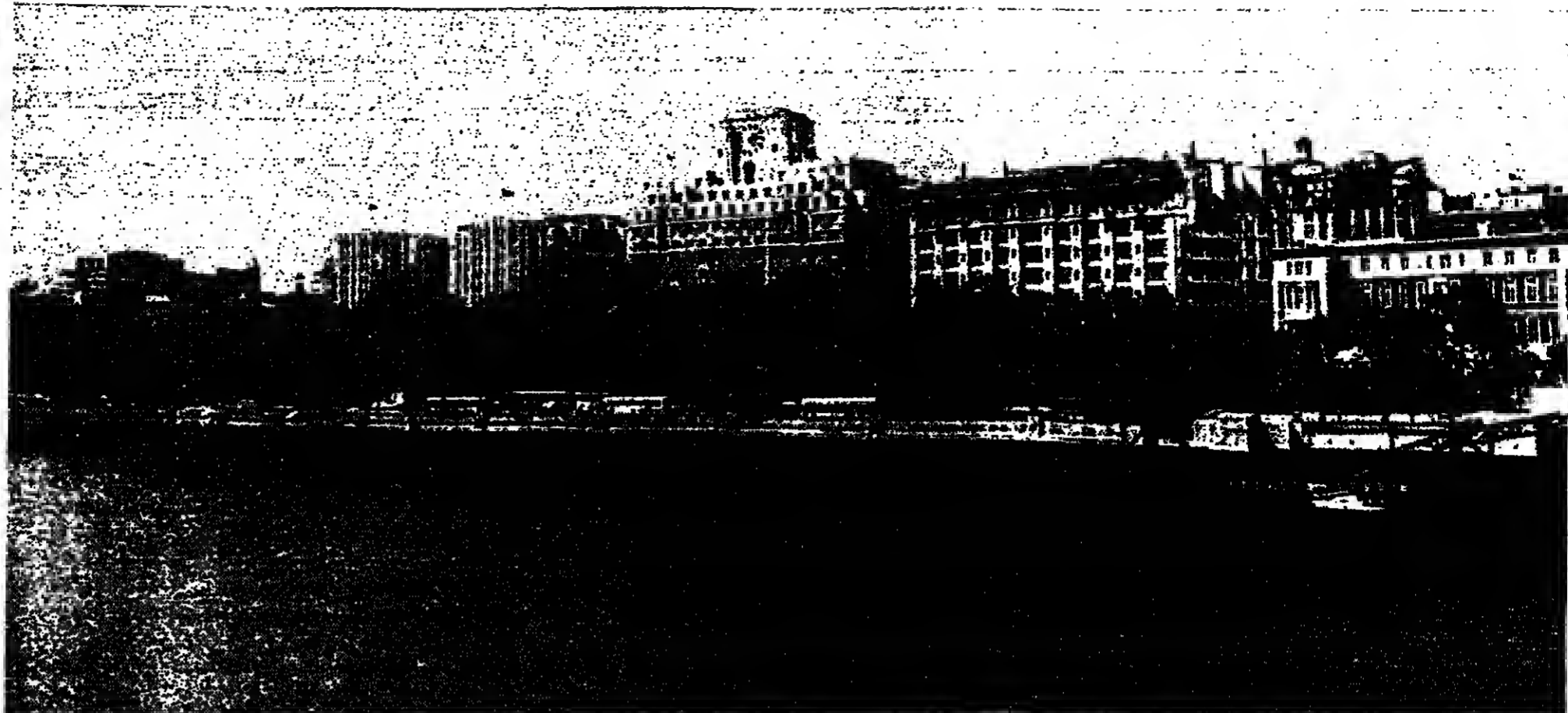
During the £85.5m renovation of Shell-Mex House in the Strand, London, by Trollope & Colls, the 1931 building has remained occupied
